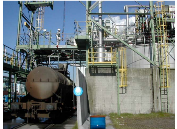
Becoflex BF Unit on a wagon loading duty
